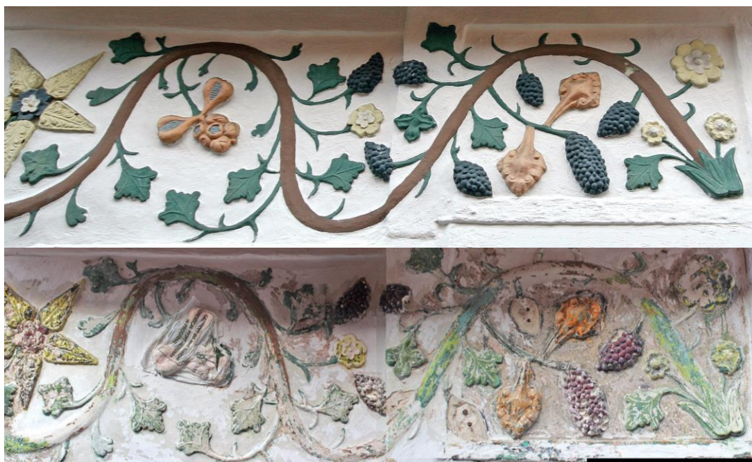
A section of the pargeting before and after the the vigorous work on the paint. The missing bunches of grapes to the right of centre are now stored. The tops of the steel pins to which they were fixed can be seen. The plaster will now have to be protected for the winter, and restored in the spring.
