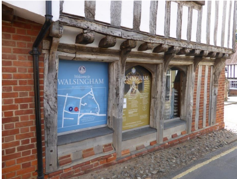
Three 15th-century shop windows on the jettied west end of 1 Common Place. (Photo by Peter Wade-Martins)
