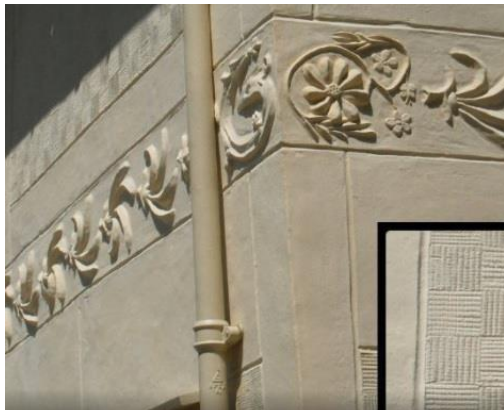
An example of Anna Kettle's original pargeting work, from www.kettlenet.co.uk
