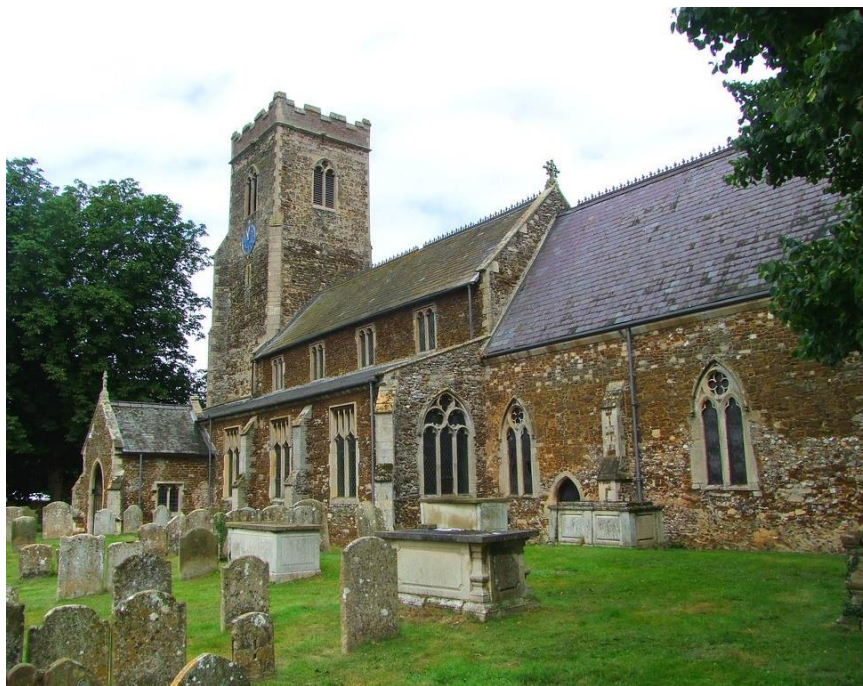
Fig 2. Middleton church, built largely of carstone. From www.norfolkchurches.co.uk , by permission of Simon Knott.
