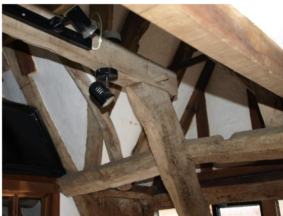
Top of truncated principal truss in south cottage
