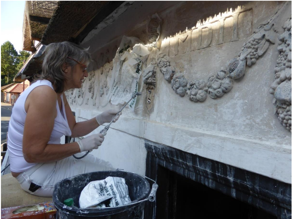
Anna Kettle about to reattach a large piece of pargeting
