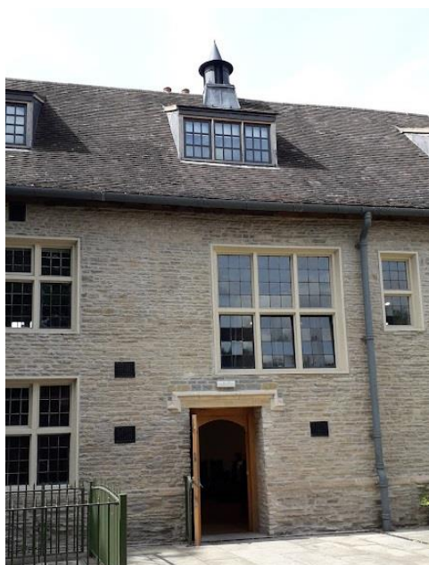
What looks like a Boyle installation at the National Civil War Centre at Newark. The cowl sucked air out of the building, and the inlet vents in the walls are helpfully picked out in black!
