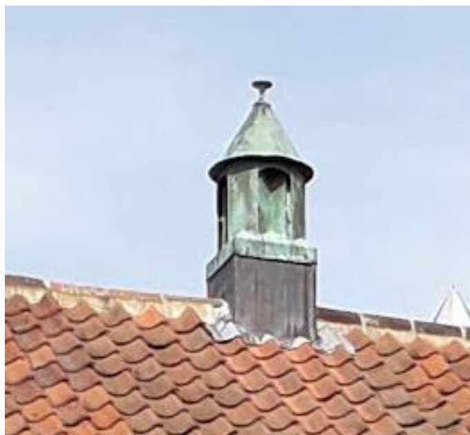
What looks like a Boyle installation at the National Civil War Centre at Newark. The cowl sucked air out of the building, and the inlet vents in the walls are helpfully picked out in black!
