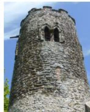
The belfry window with strip-work above it at Bessingham - below it is a bricked-up loop with a monolithic head carved from a block of conglomerate
