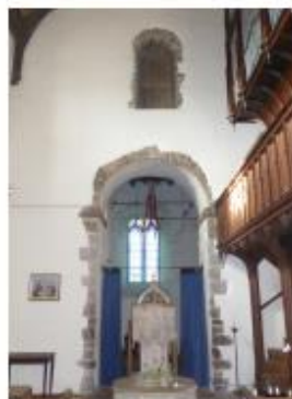
Yaxham - An impressive example of a tower arch made from a finer grained conglomerate, as well as the doorway above.
