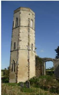
Edgefield tower with conglomerate quoining
