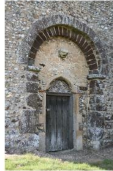
Little Snoring church Conglomerate in the tower arch of the first church The west wall of the nave of the later church showing a course of conglomerate at the base and the quoins
