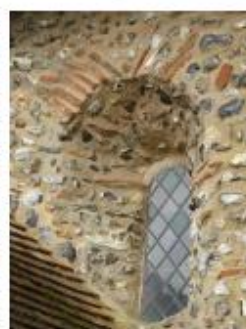
Roman tiles forming a double-splayed nave window at West Barsham
