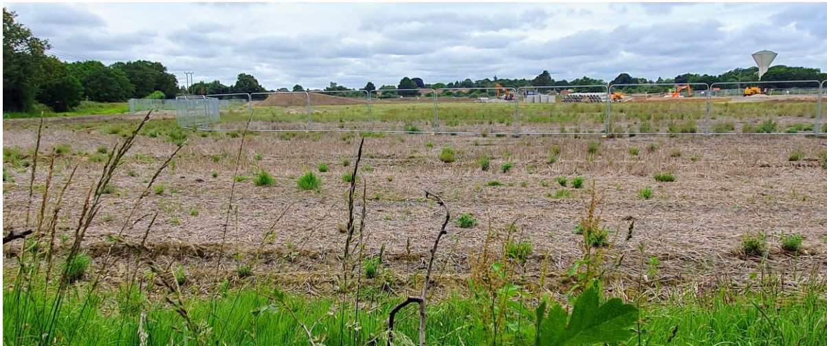
Fig 2. View of the site in early July 2024, with house-building beginning. The photograph is taken from the Restricted Byway along the east side of the site, at point X on Fig. 1, looking west across excavation Area 2, where the Roman pottery and ditches were found. Dereham's water-tower can be seen on the right and the trees on the left are on Neatherd Moor.
